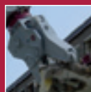
Dedicated Demolition Line
